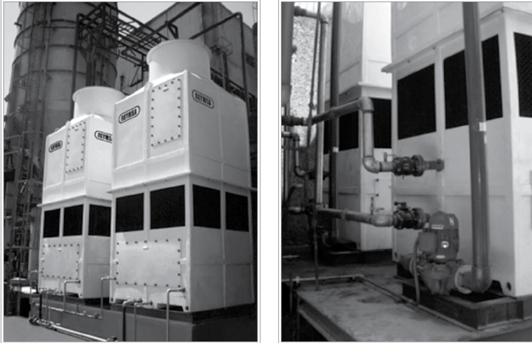
Figure A-63: Example of a base support (provided by others)
