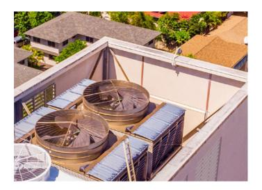
**Over time**, the engineering and maintenance teams at the Hawaii Convention Center had become frustrated with the expenses required to replace damaged parts and **corroded towers** in a short period of time, due to the **salt air environment** which destroys the towers at a much faster rate than the norm.
