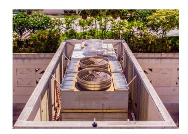
By going to FRP construction the customers now have confidence in knowing they will experience significantly lower maintenance costs, eliminate the coating expenses for the life of the tower, and they will have a cooling tower with a life expectancy of 30+ years.
